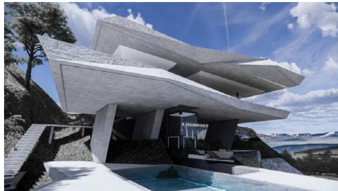
Figure 26. Fair-faced concrete is used to respond to the natural stone texture
